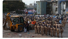
Bandra Demolition Drive 60% Complete; Stone...
